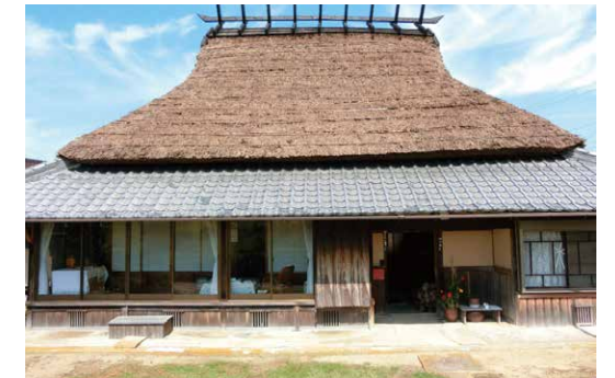
Preservation and utilization of historical structures
