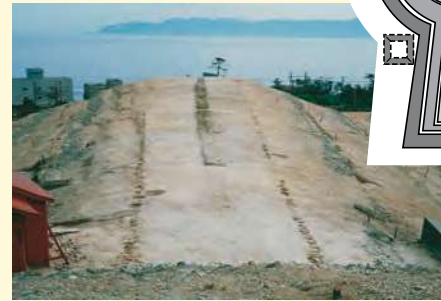
⑤The view of the front mound under digging research work
