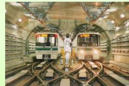
Municipal Subway Kaigan Line <Yumekamome>
